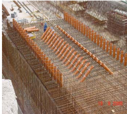
More complex: Filling through the bottom
