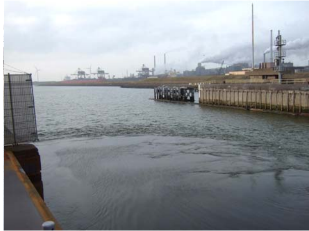
Observed salt exchange in IJmuiden
